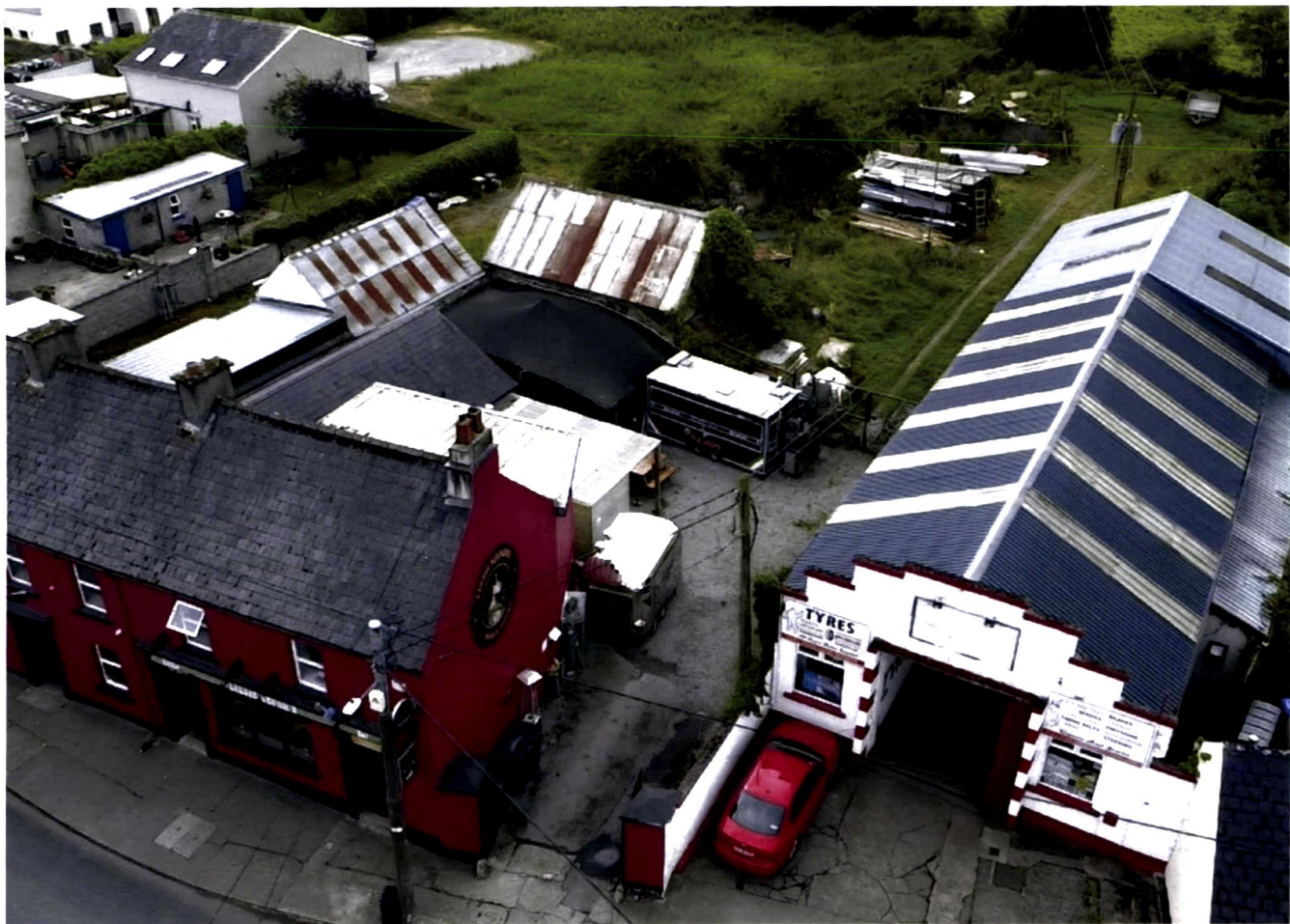
Aerial shot from Road side
